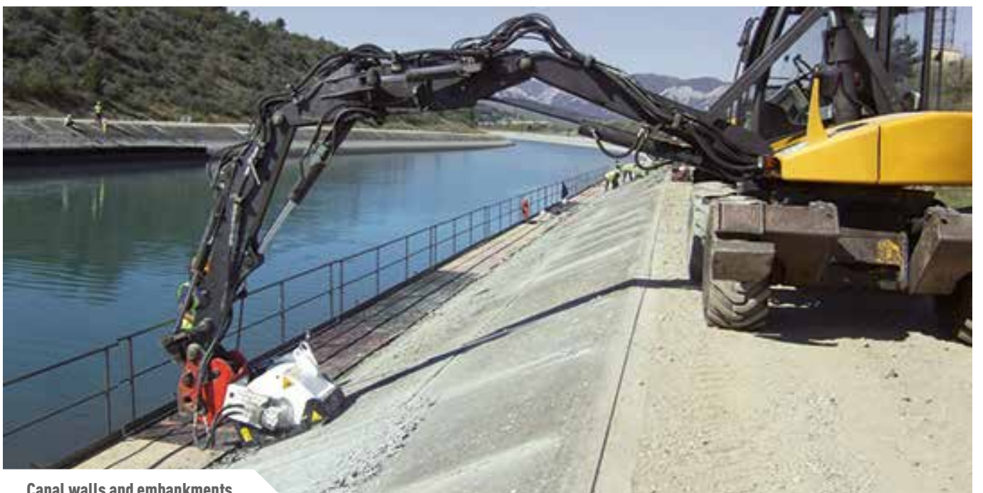
Canal walls and embankments
